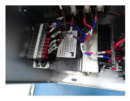
*Figure 2-9* Control transformer connection (104017-165)
