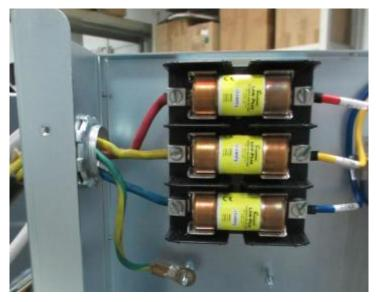
Figure 2-7 Mains cable connection
