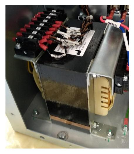
Figure 2-10 Control transformer connection (104017-162)
