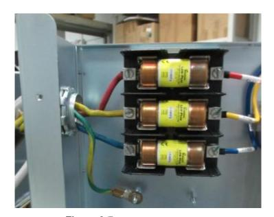
Figure 2-7 Mains cable connection
