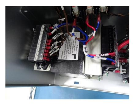
Figure 2-11 Control transformer connection (104017-165)
